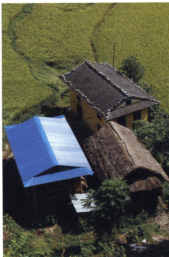
Photo 4: Different roof materials (painted corrugated galvanized iron, straw, slate) and typical building types in Rukum (Photo: J. ANHORN 2012)
